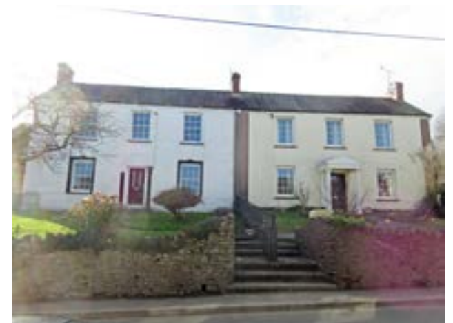
Wal gynnal o gerrig rwbel i gyrtiau blaen uwch 'Kieffe House' a 'The Kieffe'
