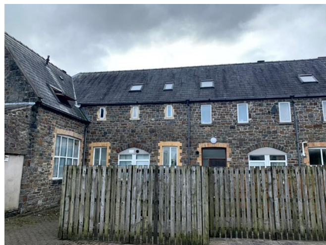
Replacement uPVC windows on the rear northeast elevation of the listed former Model School
