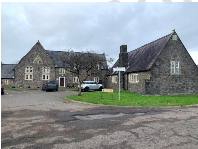
The former Model School complex north of St Catherine Street.
