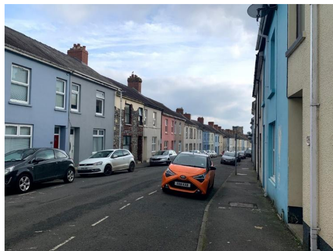
The house with removed render within the context of Parcmaen Street.
