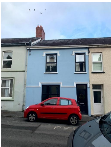
A terraced house on Parcmaen Street with additional plasterwork detailing to the window and door openings
