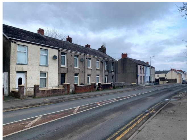
The short terraces on St Catherine Street, looking northeast, with low boundary walls and some iron railings.
