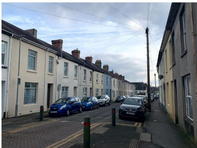
Telephone wires and TV aerials visible on Parcmaen Street.
