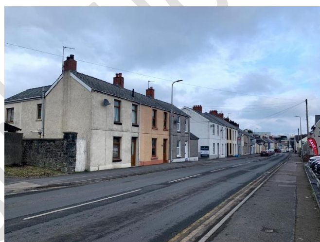
View of St Catherine Street, looking northeast
