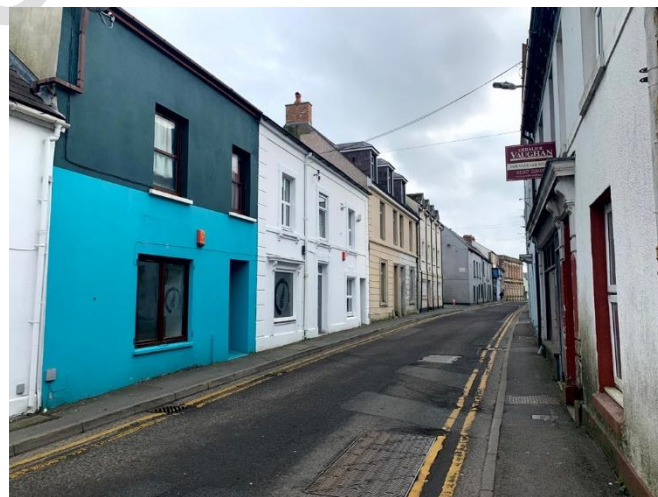
The southern half of Water Street, looking southeast. Roofs vary in height but have matching pitches and are covered in slate, whilst some of the larger building have additional dormers and rooflights to the attics.
