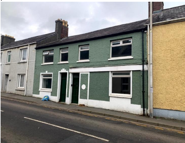
A former historic shopfront, infilled to convert the building into residential housing
