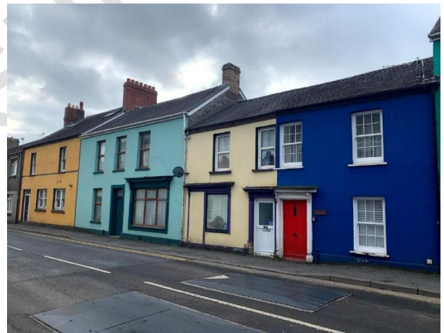
Surviving historic shop windows and timber door canopies constructed in timber.
