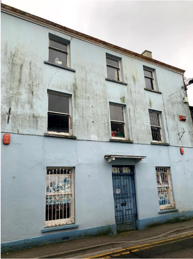
The listed building on Water Street, to which the forecourt railings of Capel Heol Dŵr are attached.
