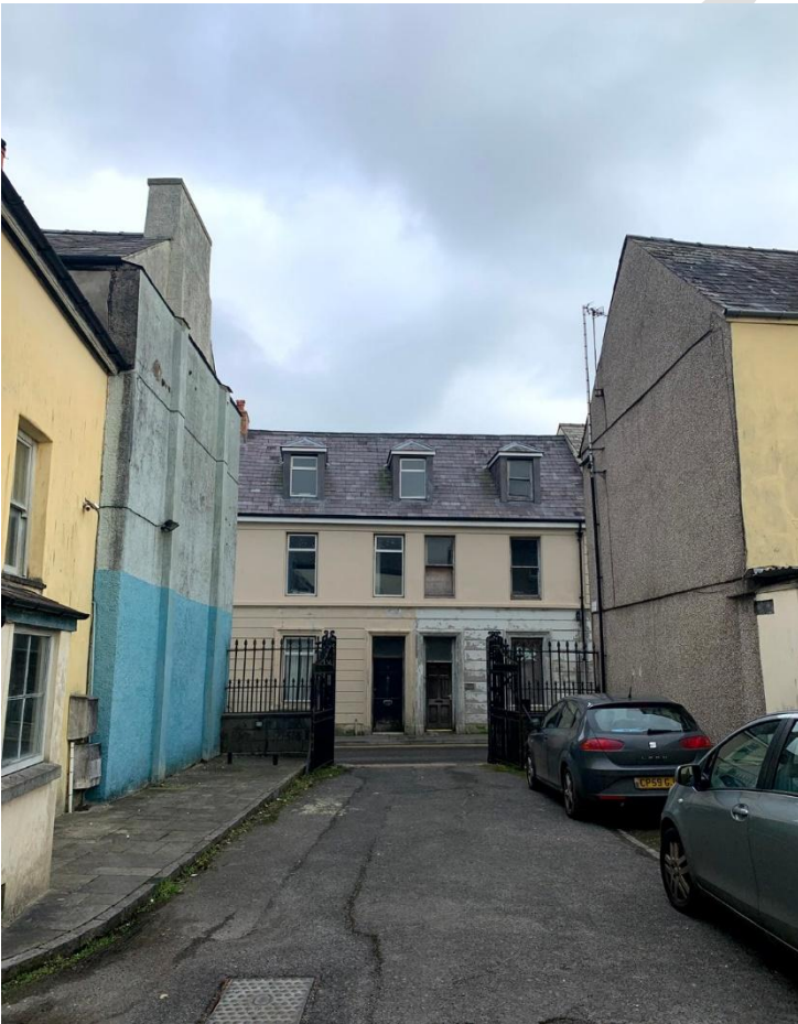
The railings and gates to Capel Heol Dŵr which separates the forecourt from Water Street.
