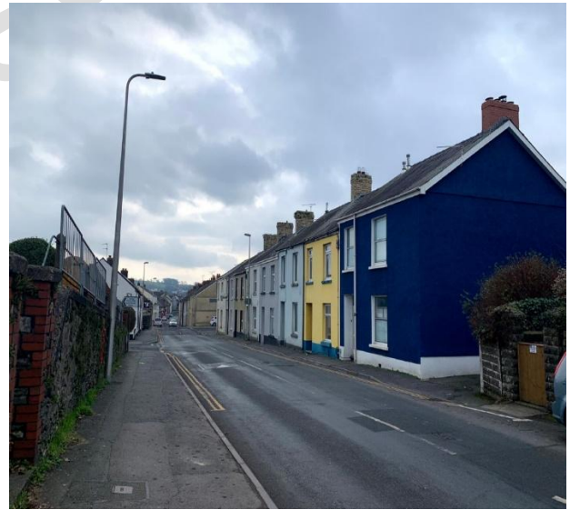
View from the Conservation Area Boundary at the north end of Water Street, looking south.
