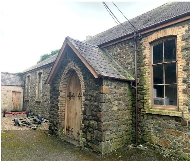
The east elevation of the Sunday School behind Capel Heol Dŵr
