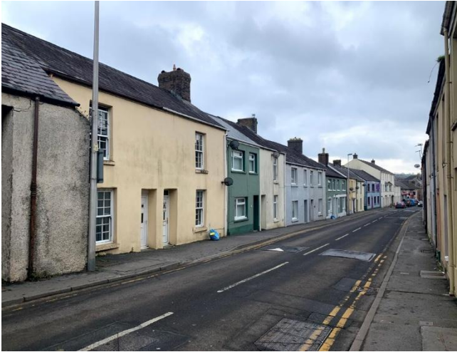
The north end of Water Street, looking southeast. Historic timber windows and doors have been replaced with uPVC units.
