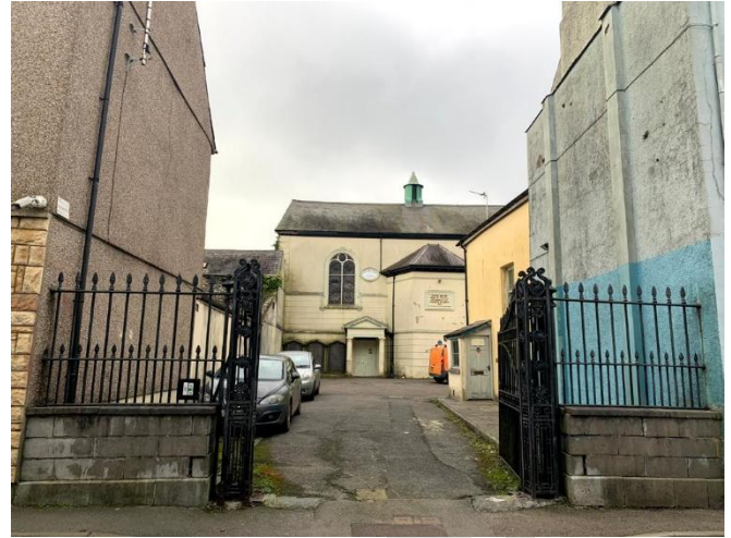
The Capel Heol Dŵr and its gated forecourt as seen from Water Street, looking west
