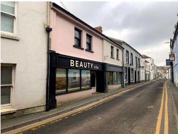
Traditional shopfronts constructed in timber.
