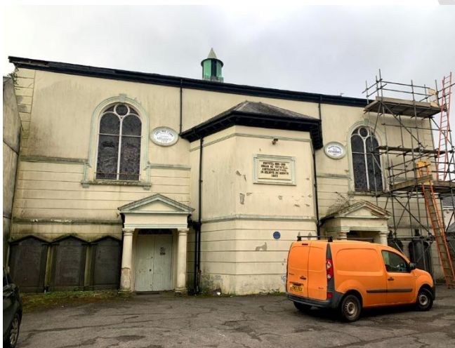
The east elevation of Capel Heol Dŵr.
