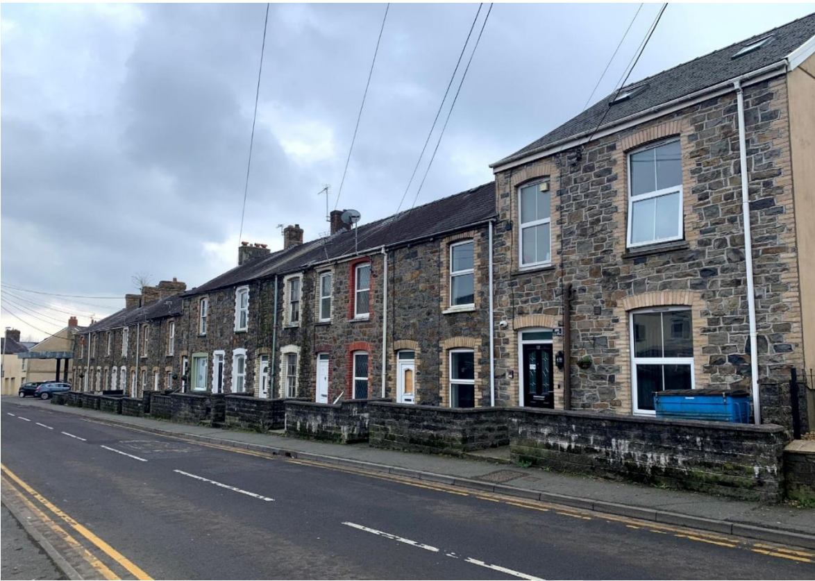
The terrace on Glannant Road with low boundary walls.
