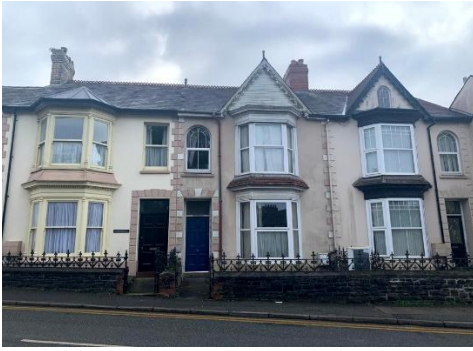
Decorative iron railings to the front forecourt of a group of terraced houses on Barn Road.
