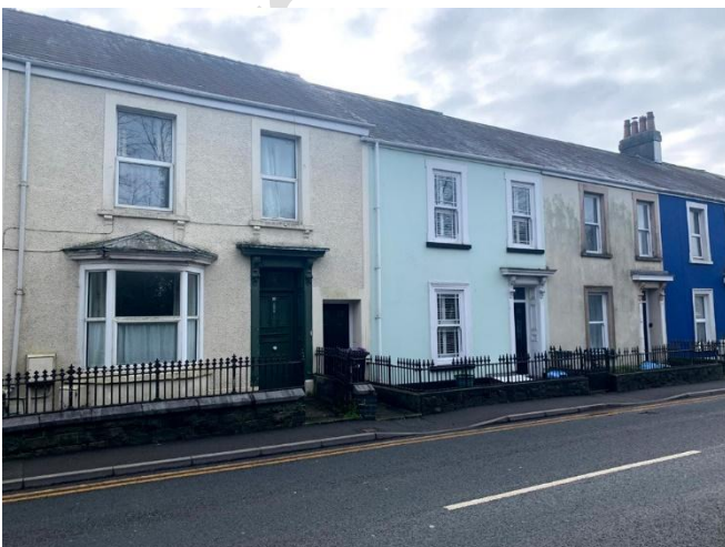
Richmond Terrace, with a variance in building size and architectural features but the common characteristic of a forecourt with historic railings.
