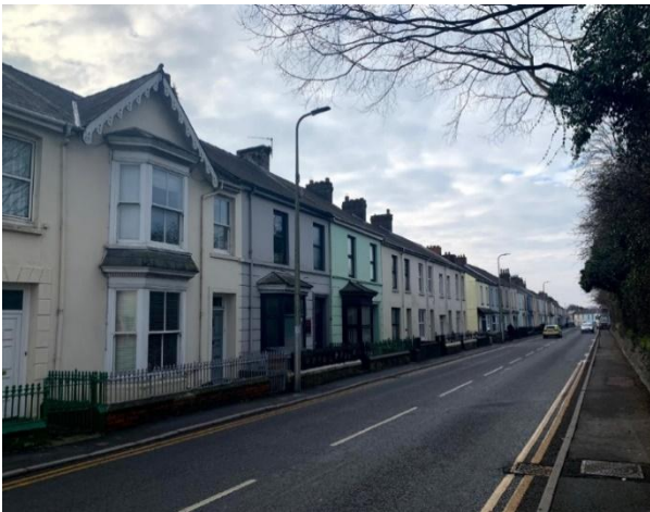
View of Richmond Terrace with Francis Terrace in the background, looking west.
