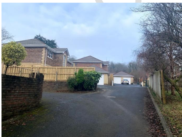
The modern development of houses east of Wellfield House
