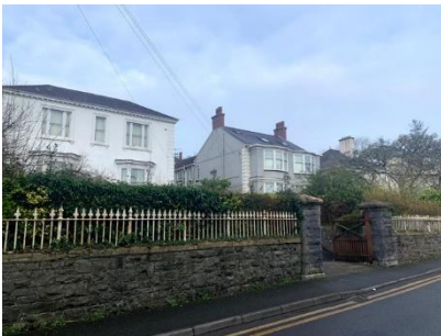
Historic iron railings on top of a rubble stone boundary wall, with accompanying gate piers to a villa on Wellfield Road
