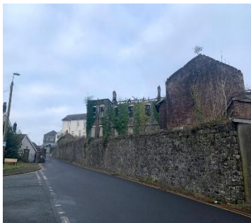
The variety of historic materials used in the construction of the former workhouse, including rubble stone and red brick.
