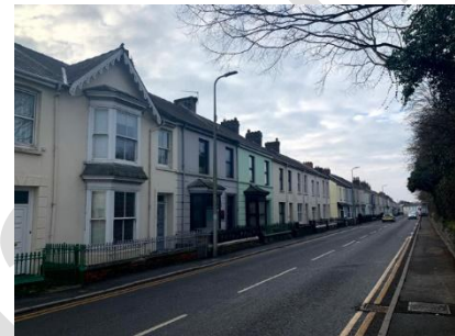
The historic iron railings to the front facades of Richmond Terrace.
