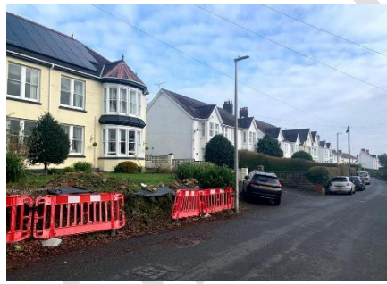
The variety of roof styles used to accommodate projecting bay windows on Long Acre Road, including gables and semi-circular turret style
