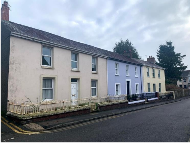
Larger terraced houses on Waterloo Terrace. The central house, Meiros Hall, is a listed building.
